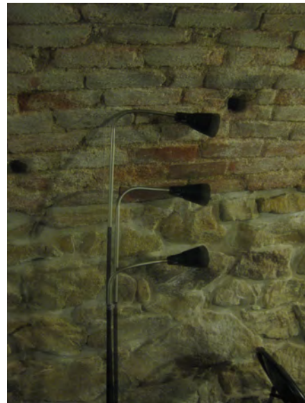
Lighting is domestic spotlights
